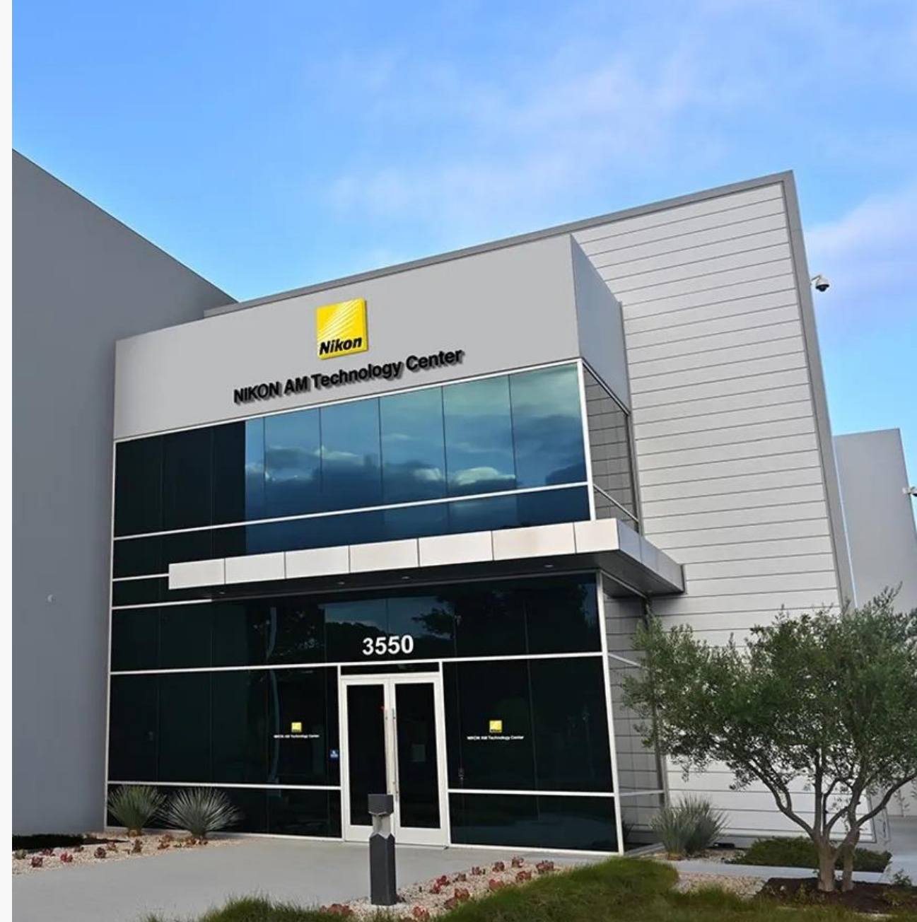
Nikon metal additive manufacturing and R&D center in Long Beach
