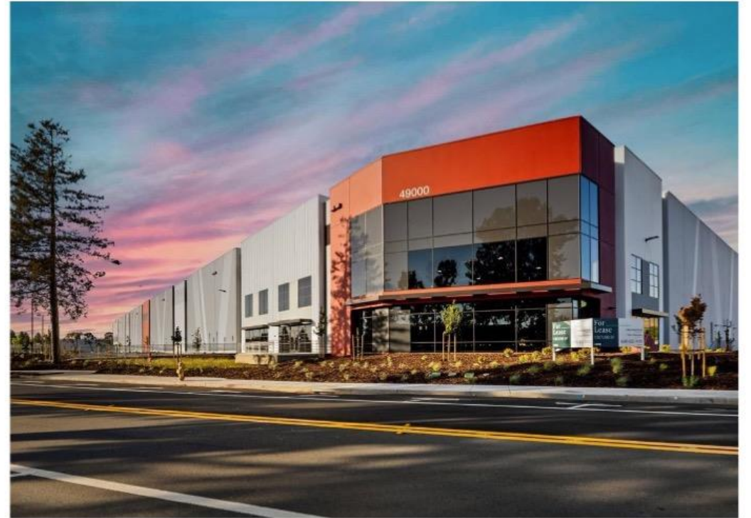
Fremont Industrial Bldg.
